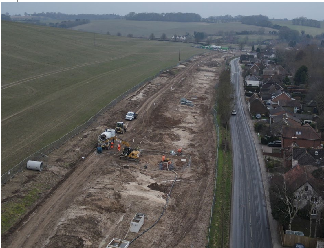
Figure 4: Drone footage halfway down the pipeline. Work on one of the manholes is visible near the vehicles in the photograph.
