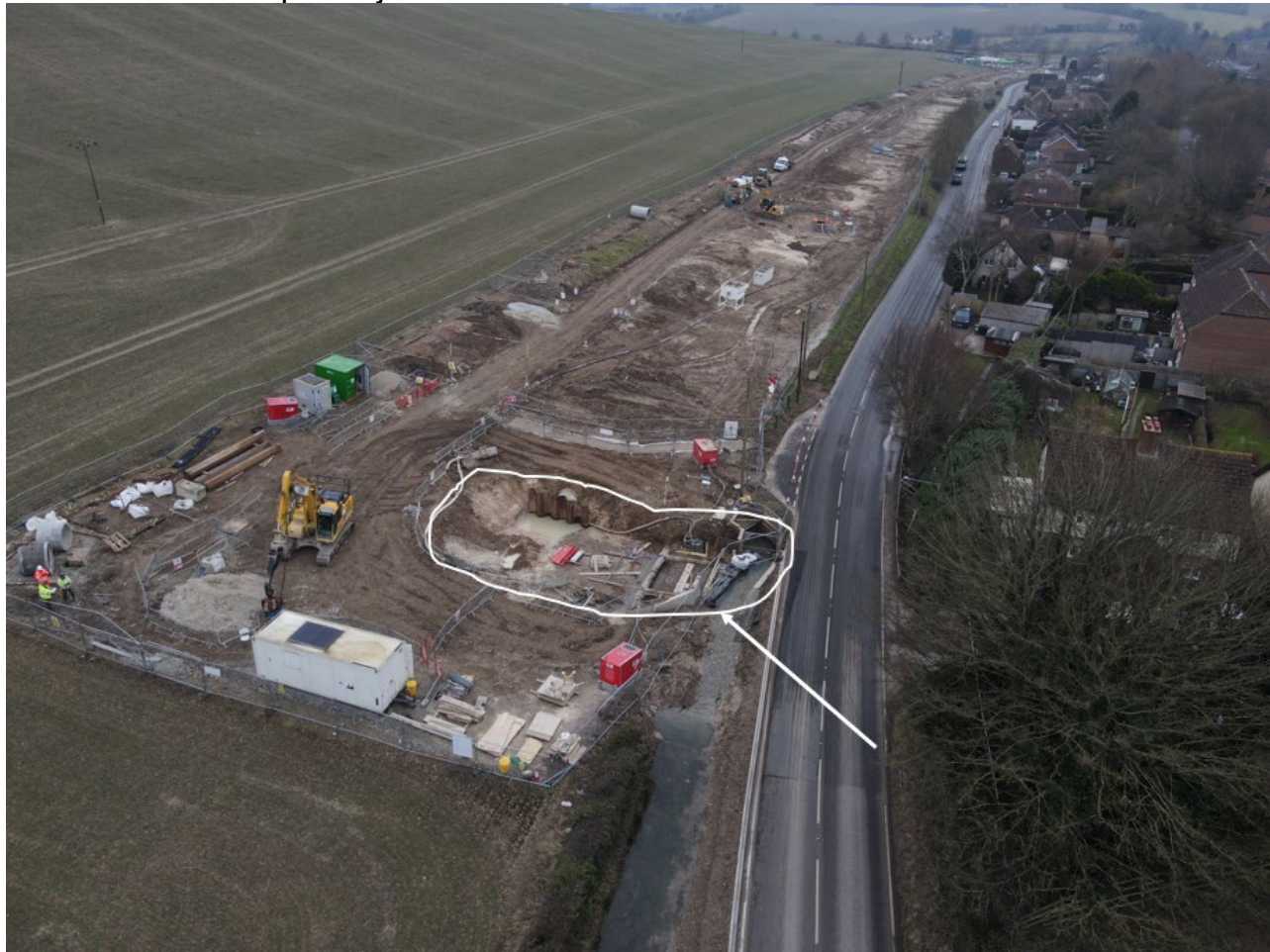
Figure 2: Looking downhill towards the River Lambourn. The construction of the offtake works is visible in the foreground (highlighted with the white arrow and outline). The drone footage was taken on 19 February 2025.
