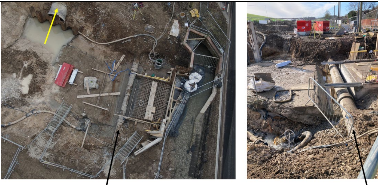
Figure 3: The left photo is drone footage taken on 19 February 2025. I took the right photo on the 25 February 2025 with progress having been made on the concrete slabs. The yellow arrow on the left shows the location of the new 1.35m diameter pipeline. The much smaller West Berkshire Groundwater Scheme pipeline is indicated in both photos using a black arrow. The offtake of the flood scheme is being constructed to pass over the older pipeline. The water in the foreground of the right photo is groundwater which continues to seep into the construction site.
