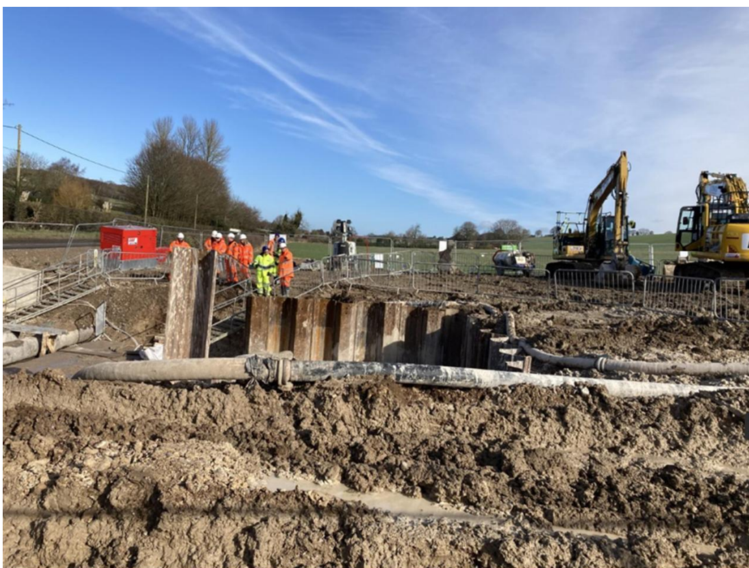
Figure 5: One final photo of the offtake area -as a reminder of some of the really tough conditions faced on site (February 2025)
