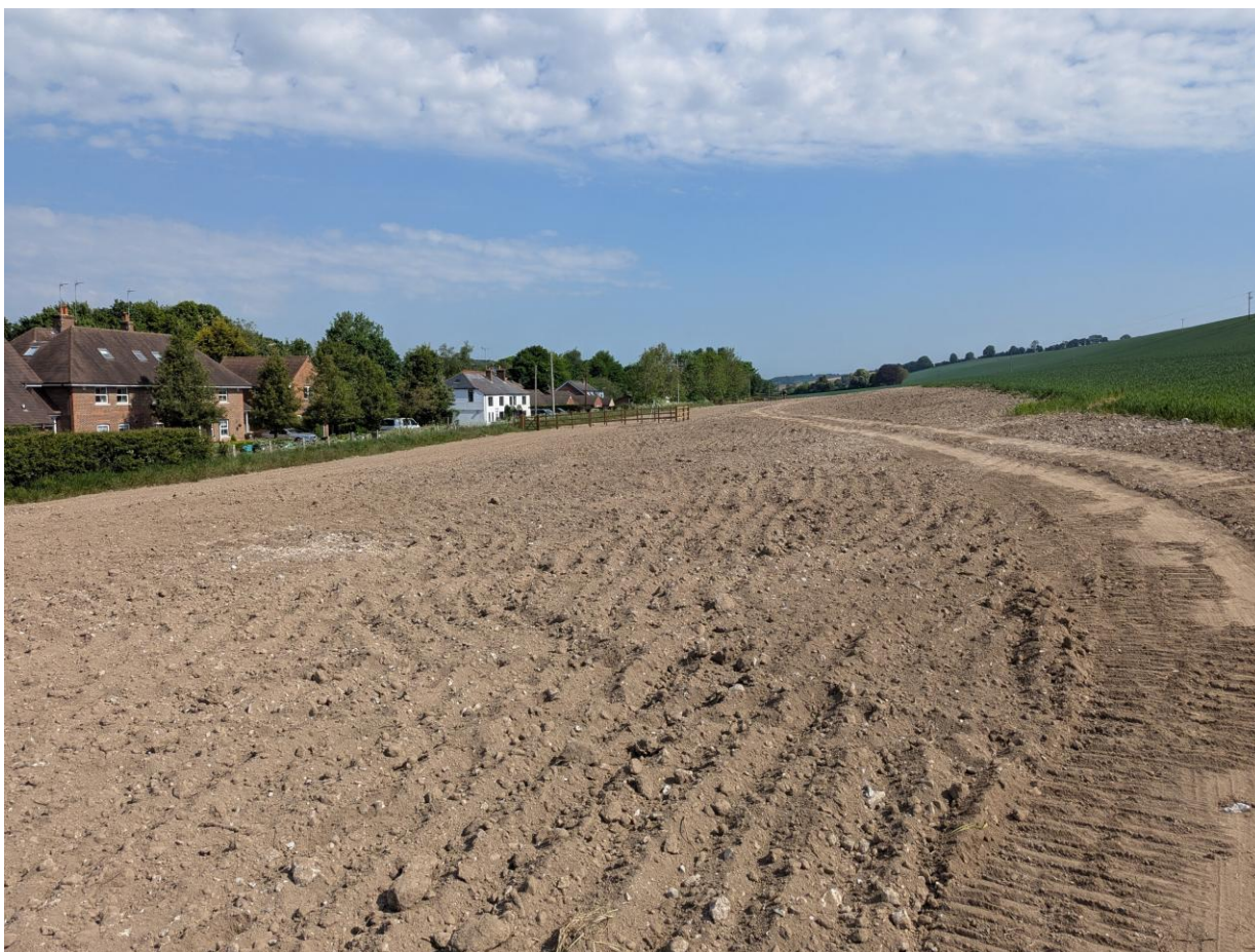
Figure 2: Looking upstream along the pipeline. The fencing in the middle distance is on of the manholes needed for maintenance. (May 2025)
