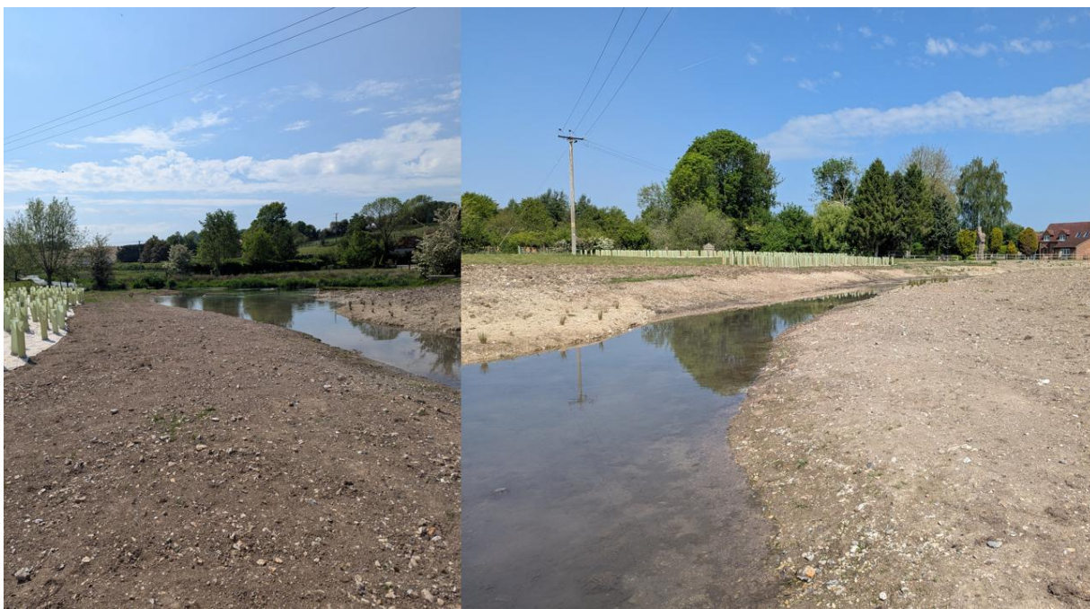
Figure 4: Left - Looking downstream near the new backwater into the river Lambourn. New planting on the left - protected in plastic sleeves. Right - Looking upstream at the new open channel. (May 2025)
