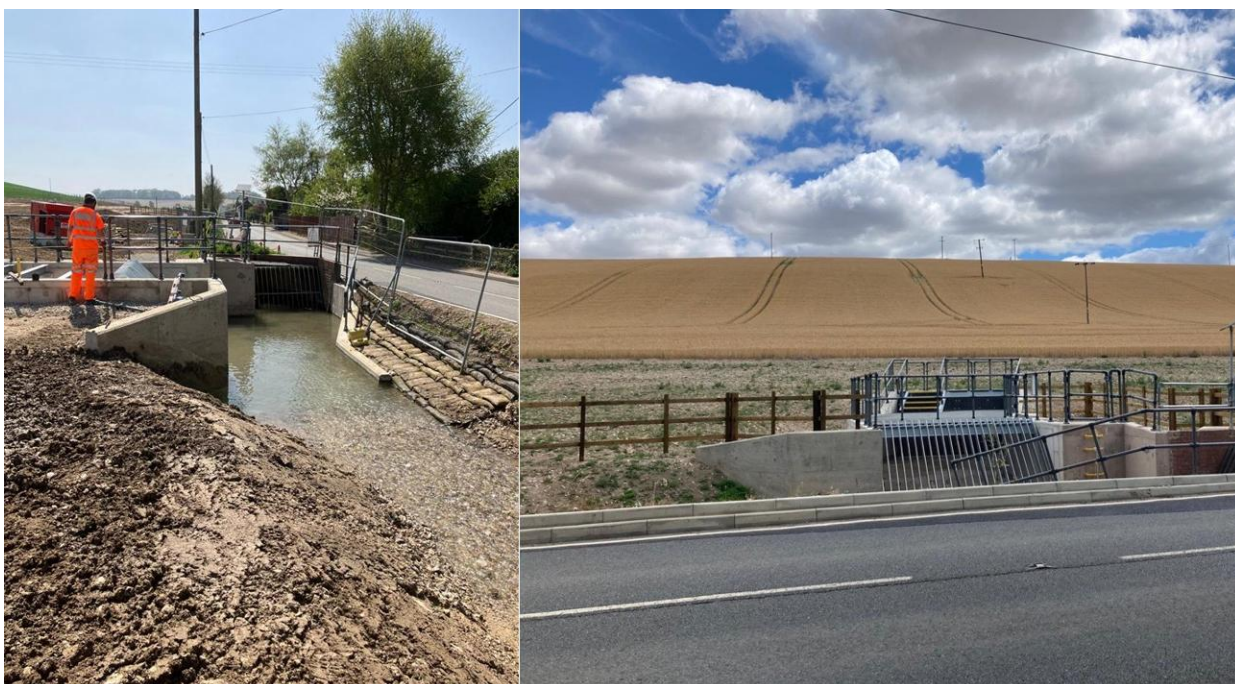
Figure 1: Left - Great Shefford Stream - looking downstream (May 2025). Right - looking towards the offtake - original culvert on the right of this photo (July 2025)
