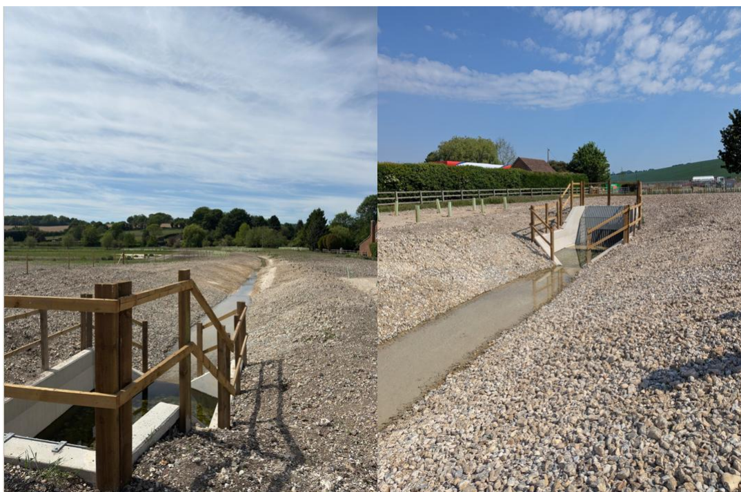
Figure 3: Left - looking downstream at the new open channel. Right - looking upstream towards the transition chamber and stilling basin. (May 2025)
